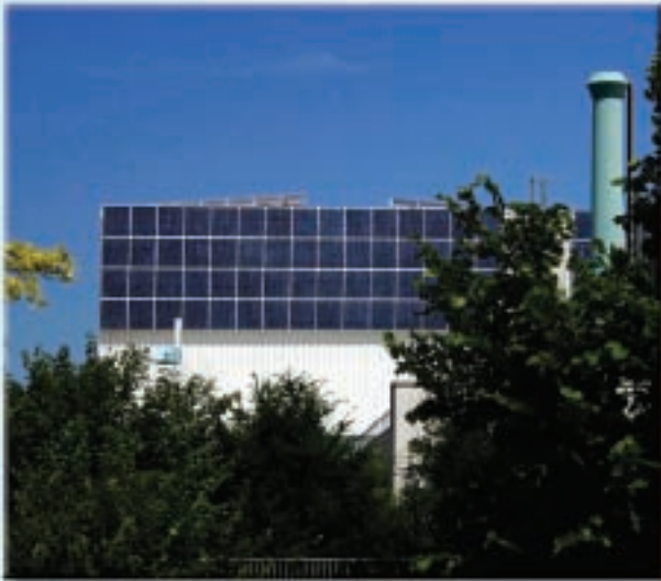
1,000 sq. meters of solar panels affixed to Dow Corning's Wiesbaden, Germany manufacturing site
