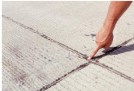
*The first installation of Dow Corning<sup>®</sup> 888 Silicone Joint Sealant in an airport is still performing well after nearly 20 years.*
