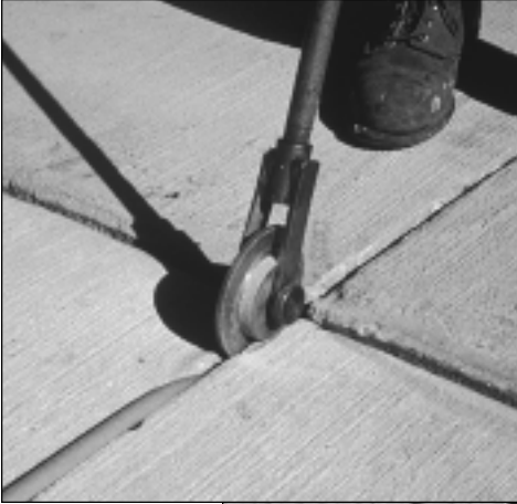
Installing Dow Corning 890-SL Self- Leveling Silicone Joint Sealant
