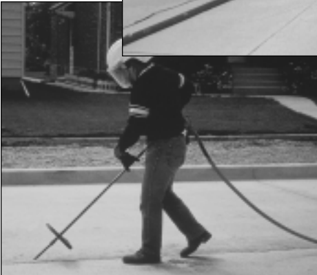
Air-blasting the joint
