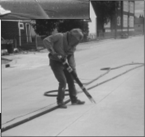
Air-blasting the joint
