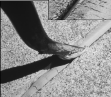
Tooling the Dow Corning 888 Silicone Joint Sealant
