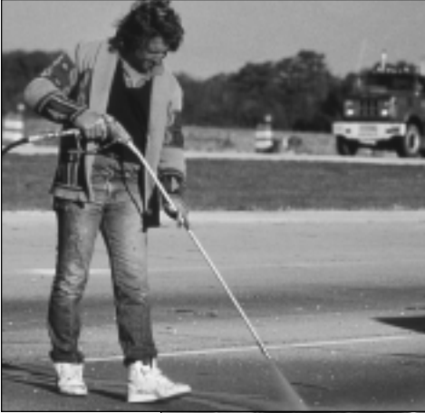
Sandblasting the joint
