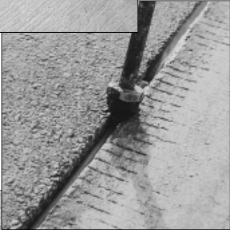
Tooling the Dow Corning 888 Silicone Joint Sealant
