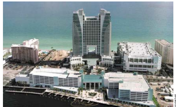
Impact-resistant glazing in rooms and suites at the new Westin Diplomat was constructed with Dow Corning ® 995 Silicone Structural Adhesive, while the flowing 6-story glass canopy used Dow Corning ® 795 Silicone Building Sealant. Perimeter joints were sealed with Dow Corning ® 790 Silicone Building Sealant, an ultra-low modulus, high-elongation material.
