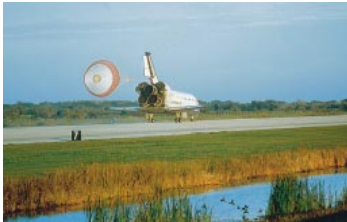
NASA chose Dow Corning® brand silicone sealants to repair the joints and pavement cracks on the 15,000-foot shuttle landing strip. Photos by NASA.
