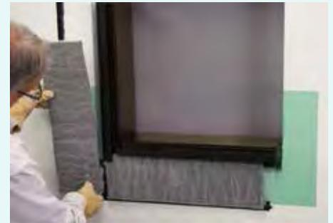
3. Firmly press the blanket to the wall to ensure good contact of the sealant to the substrates.
