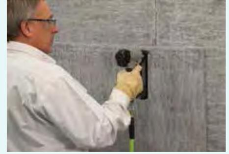
1. Apply a bead of *Dow Corning* weatherproofing sealant to the *Dow Corning* Building Insulation Blanket.
