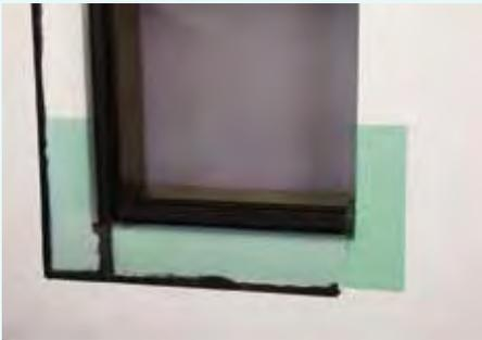
1. Install window-curtainwall transition materials – including the *Dow Corning* Silicone Transition System and *Dow Corning* 778 Liquid Flashing – as required.
