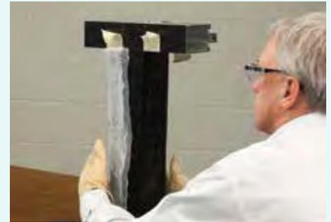
3. Firmly apply the *Dow Corning* Building Insulation Blanket to the mullion to ensure good adhesion.
