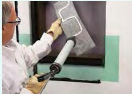
2. Apply a bead of *Dow Corning* weatherproofing sealant to the *Dow Corning* Building Insulation Blanket.
