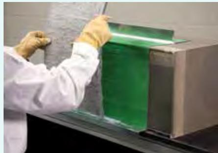
2. Firmly press the blanket to the slab edge to ensure good contact of the sealant to the substrates.
