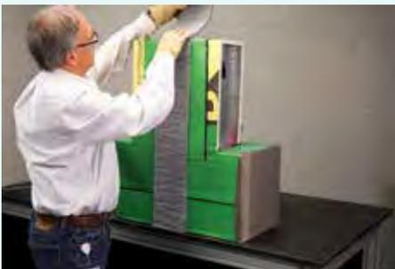
4. Crease a sharp corner fold into the insulation blanket to ensure optimum aesthetics and fit.
