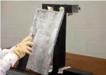
1. Apply spray adhesive to the back side of the *Dow Corning* Building Insulation Blanket.
