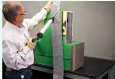
2. Apply a bead of *Dow Corning* weatherproofing sealant to the *Dow Corning* Building Insulation Blanket.
