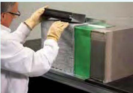
4. Continue with curtainwall installation using standard construction techniques.
