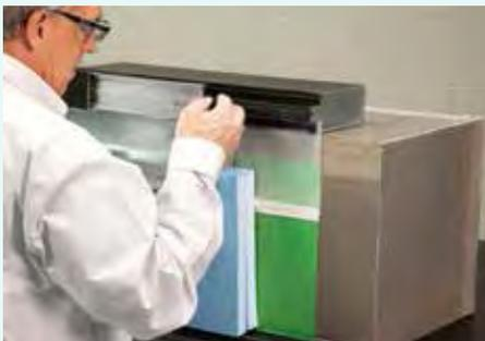
4. Apply flashing over the insulation blanket using standard installation techniques.
