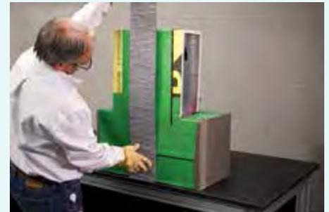
3. Firmly press the blanket to the wall to ensure good contact of the sealant to both substrates.
