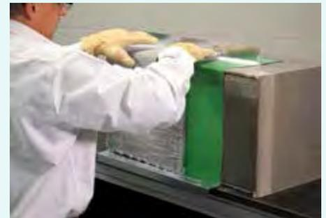
3. Secure the insulation blanket, ensuring a sharp corner fold for best fit.
