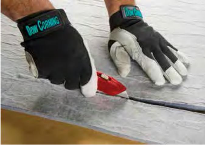
Cutting Dow Corning® Building Insulation Blanket with a utility knife.
