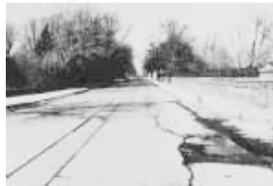
*The 60-year-old concrete pavement past Newport’s famous mansions was dangerously cracked and worn before it was replaced with materials that echoed the original.*
