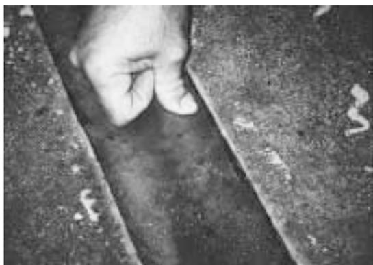
*Three types of Dow Corning® brand silicone joint sealants are being used to seal concrete pavement joints like this one in both new and remedial applications throughout the City of Ft. Worth, Texas.*
