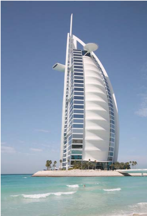
Figure 1. Burj-Al-Arab Hotel, Dubai; a tribute to the use of structural glazing silicone adhesive in a high-rise façade.
